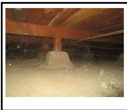
Pictures 1 thru 3... The crawl space soil was dry during this inspection, the flooring supports and sub flooring were in acceptable condition.
