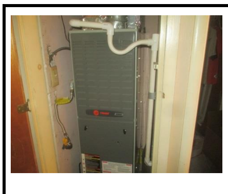
Picture 1... The gas fired forced air heating system was in acceptable working condition.
