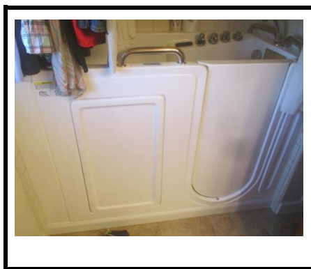
Pictures 1 thru 3... The hall bath walk in jetted tub was operated and in acceptable working condition, the motor compartment was in acceptable condition with no signs of leaks, the GFCI protection resets are located in the hall bath closet.
