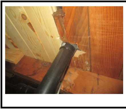
Pictures 1 thru 3... The sub flooring under the master bath shower, toilet and hall bath toilet was in acceptable condition with no leaks or damage observed.
