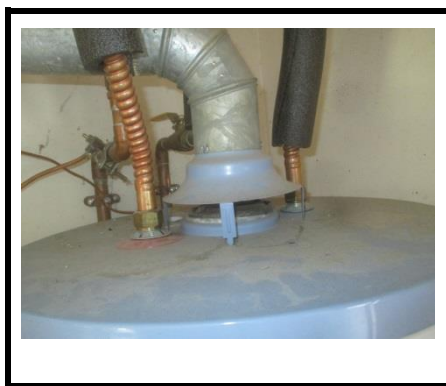
Pictures 1 thru 3... The water heater was in acceptable working condition with no leaks or damage observed.
