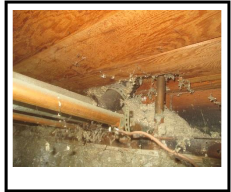
Picture 1... The sub flooring under the hall bath jetted tub was in acceptable condition with no leaks observed.
