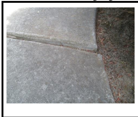
Picture 1... The uplifted section of concrete at the right front corner of the house causes a trip hazard.
