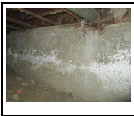
Pictures 1 thru 3... The concrete foundation walls were in acceptable condition with no significant cracks observed however some minor efflorescences observed and one chipped out area under the back slider door ,leaving the steel rebar exposed, the exposed steel rebar should be sealed or coated with anti corrosion mastic.
