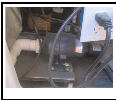
Pictures 1 thru 3... The hall bath walk in jetted tub was operated and in acceptable working condition, the motor compartment was in acceptable condition with no signs of leaks, the GFCI protection resets are located in the hall bath closet.
