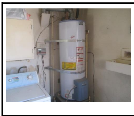
Pictures 1 thru 3... The water heater was in acceptable working condition with no leaks or damage observed.
