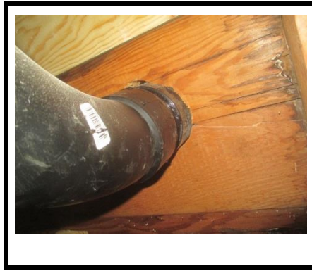
Pictures 1 thru 3... The sub flooring under the master bath shower, toilet and hall bath toilet was in acceptable condition with no leaks or damage observed.
