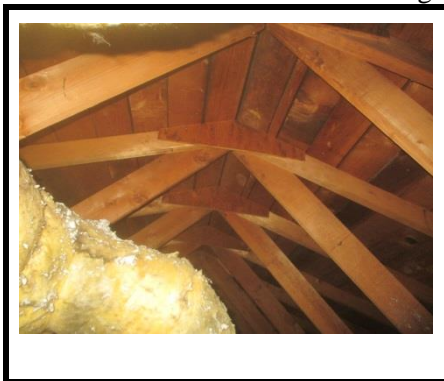
Pictures 1 thru 3... The attic area and roof framing were in acceptable condition and well insulated. The attic area in the garage was in acceptable condition however the firewall between the garage and the house was open in one area, sealing up the firewall is recommended.
