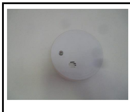
Pictures 1 & 2... The carbon monoxide and smoke detectors did respond when the test buttons were pushed.
