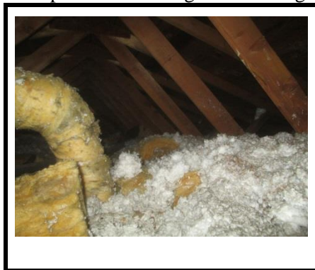
Pictures 1 thru 3... The attic area and roof framing were in acceptable condition and well insulated. The attic area in the garage was in acceptable condition however the firewall between the garage and the house was open in one area, sealing up the firewall is recommended.
