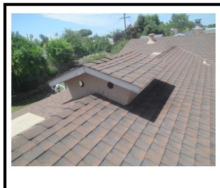
Pictures 1 thru 3... The asphalt composition roof covering was in acceptable condition, the pop up top is decorative only.
