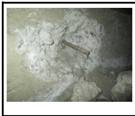
Pictures 1 thru 3... The concrete foundation walls were in acceptable condition with no significant cracks observed however some minor efflorescences observed and one chipped out area under the back slider door ,leaving the steel rebar exposed, the exposed steel rebar should be sealed or coated with anti corrosion mastic.
