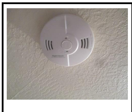
Pictures 1 & 2... The carbon monoxide and smoke detectors did respond when the test buttons were pushed.
