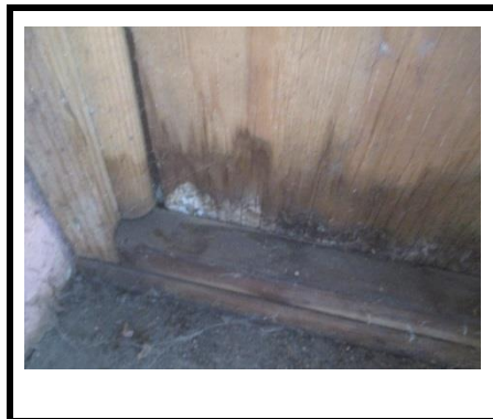
Pictures 1 thru 3... The attached storage shed at the right side of the house had several areas of fungus damage observed.
